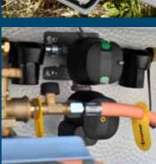
Gas changeover regulator automatically switches over to the spare bottle when the first runs out.
